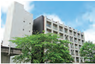
生物棟 (青葉山) Biology Building (Aobayama Campus)
